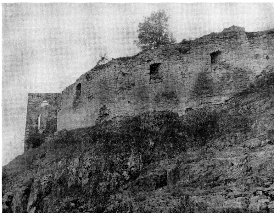
11. Tuff-wall with loop-holes in front of the gun-emplacement (16. century).
