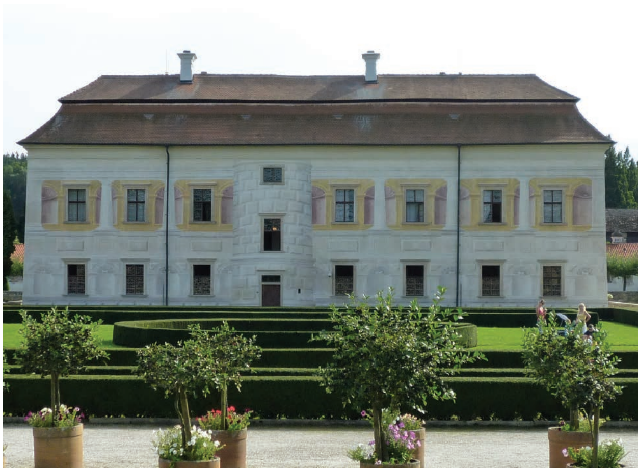
8 – View of the back façade of the central villa and its fictitious painted bastion (“staircase tower”)
