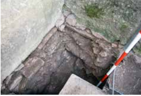
Obr. 6. Sonda S2/11 – cezúra v základovom murive medzi loďou a vežou kostola. Foto A. Balogh. Fig. 6. Test pit S2/11 – gap in the masonry foundations between the nave and the church tower. Photo A. Balogh.
