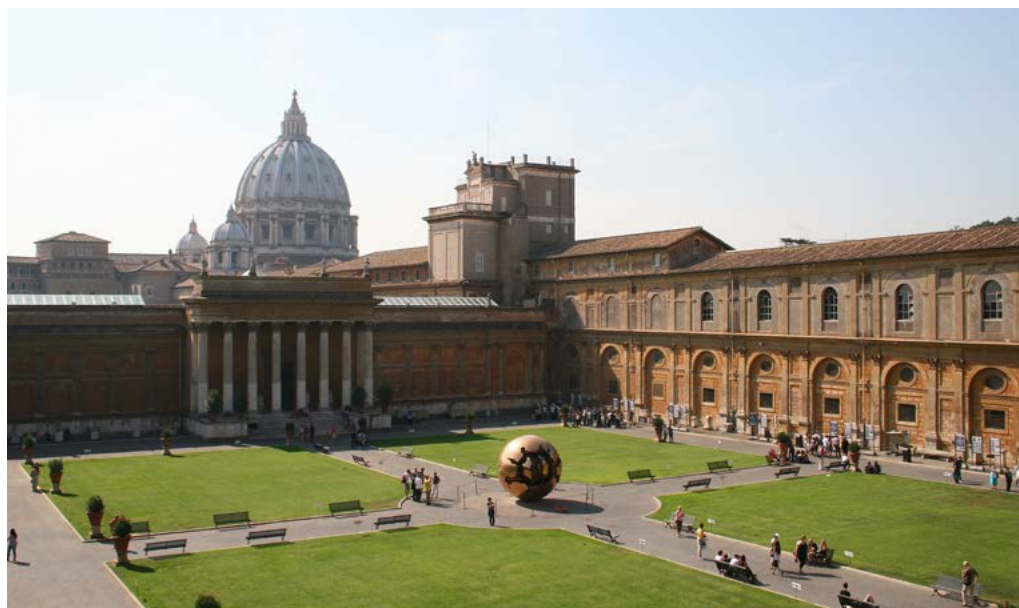
Figure 3: Courtyard of the Pinecone (Cortile della Pigna), view towards the Braccio Nuovo (with a columned portico).
